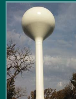
Elevated Water Storage Tank
