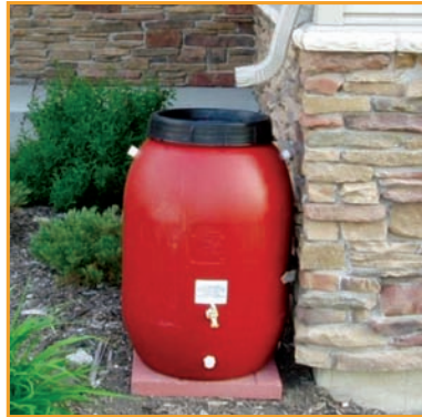
Rain barrels can reduce, or eliminate, potable water use for landscaping irrigation.
