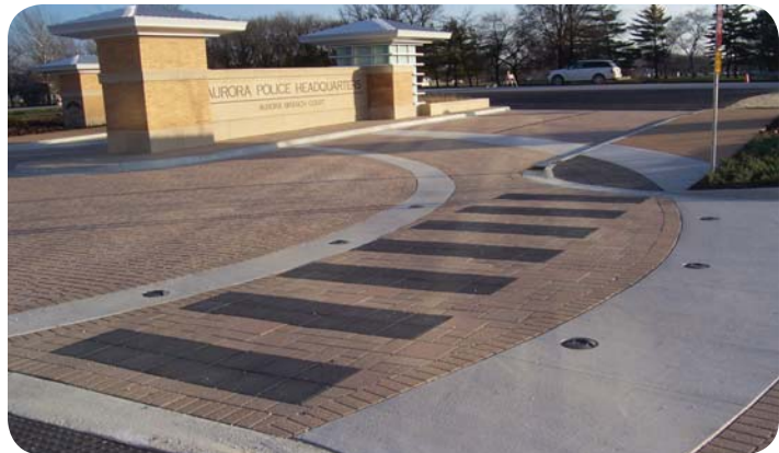
Contrasting Permeable Pavers
