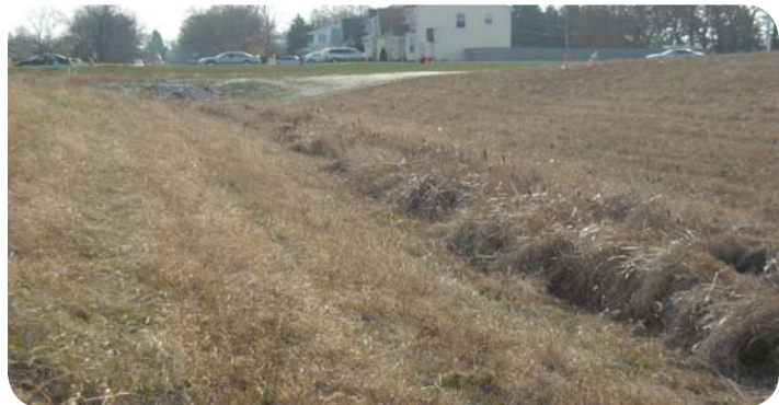
1,000 Linear Feet of Vegetative Swales
