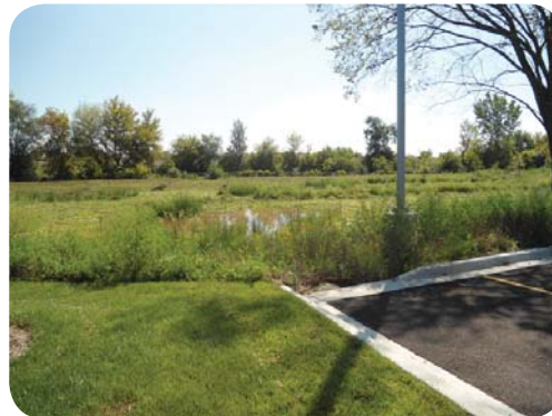
Detention Basin with Curb Flume
