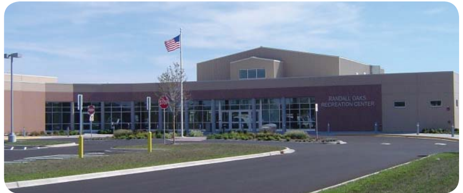
Single Story Main Entrance
