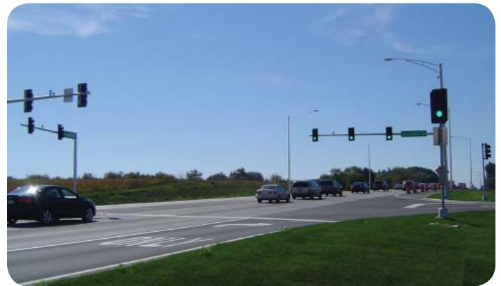
New Right Turn Lane - Randall Road to Recreation Drive
