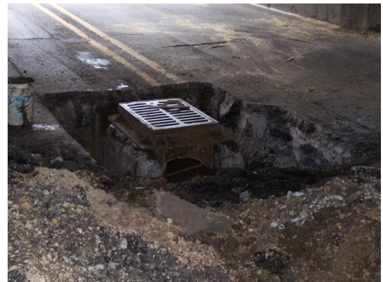
Main Street stormwater infrastructure improvements
