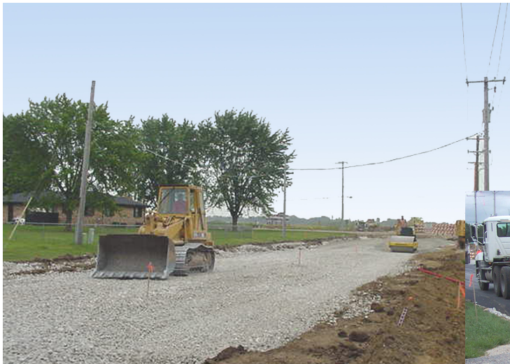
Installation of subbase
