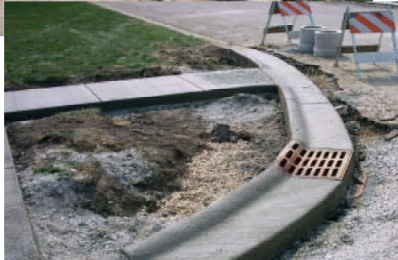
Repair of curb and gutter sections
