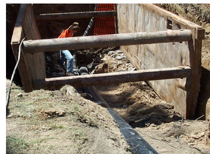
Sewer installation via pipe bursting
