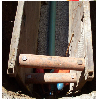
Sewer installation via open cut
