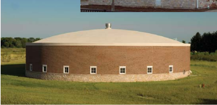
Ground Storage Reservoir
