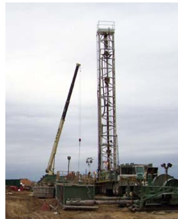
Well No. 10 Construction
