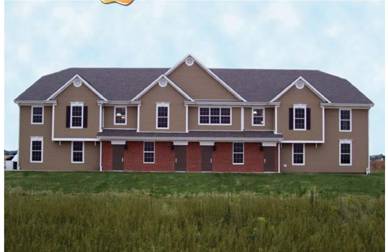
Wells No. 10 & 13 Water Treatment Plant
