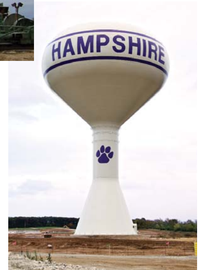
Tamm's Farm Elevated Water Storage Tank
