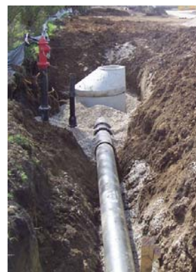
Water Main Installation
